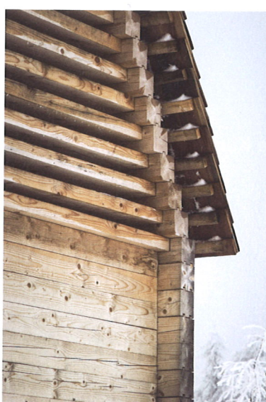
Nut-Feder-Verkämmungen Tongue and groove and comb joints
